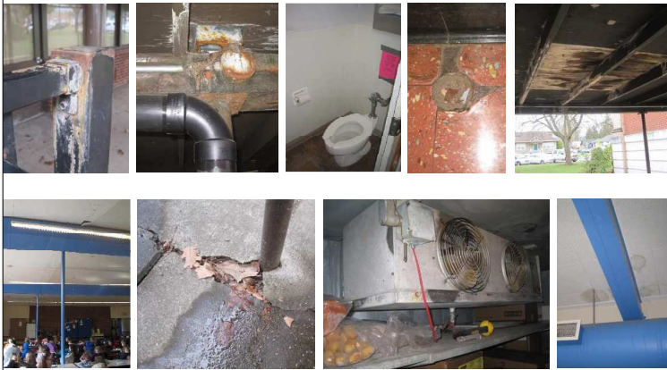
Building Condition: Edwards ES (Cafeteria)
