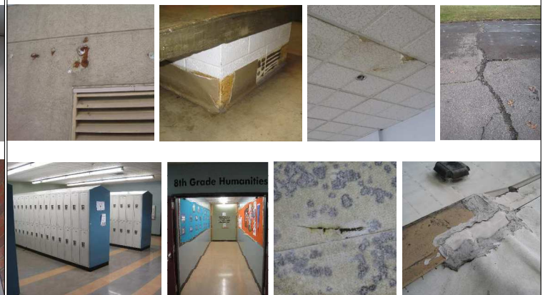
Building Condition: Mountain View MS
