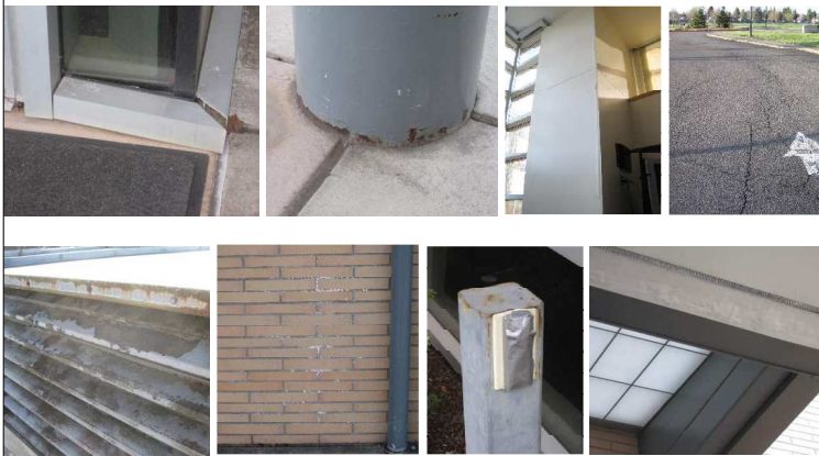
Building Condition: Joan Austin ES
