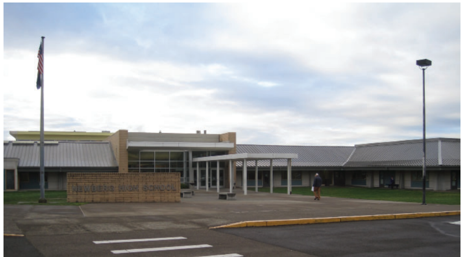
Newberg High School - Main Building (A-G): Exterior View
