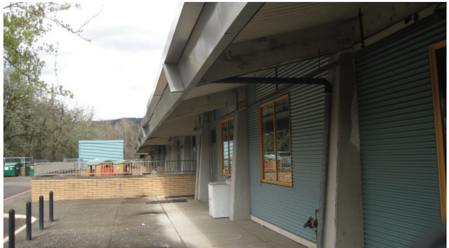
Newberg High School - Building J (CTE): Exterior View
