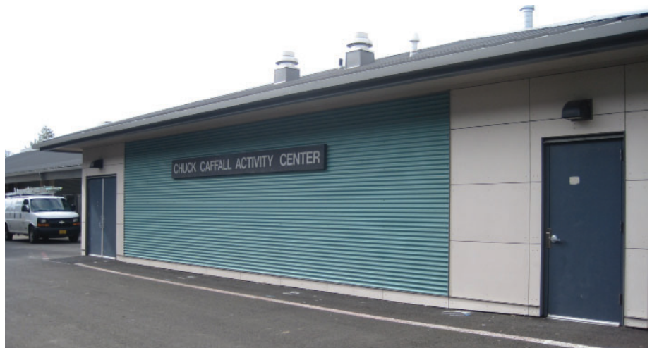
Newberg High School - Building M: Exterior View
