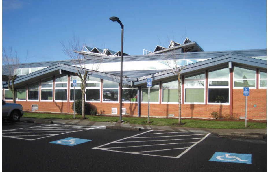
Mabel Rush Elementary School: Exterior View
