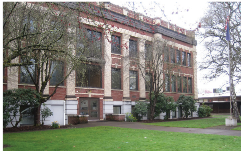
District Office: Exterior View
