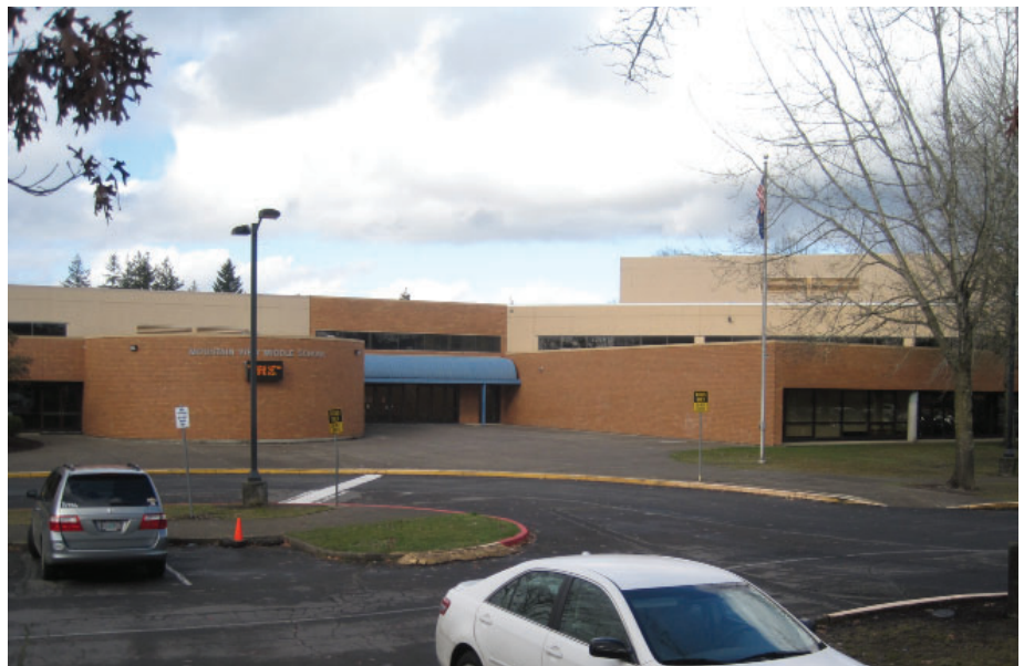
Mountain View Middle School: Exterior View
