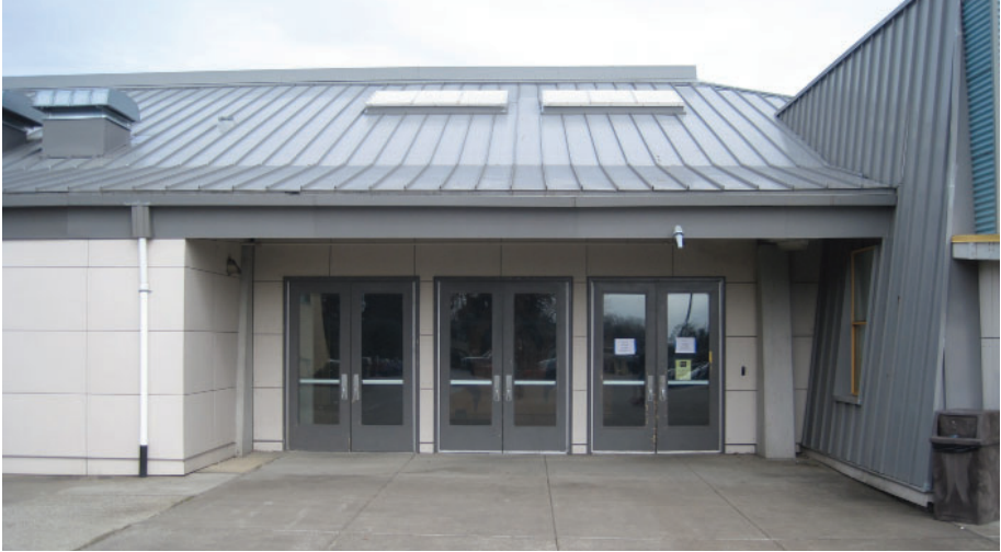
Newberg High School - Building N (Main Gymnasium): Exterior View
