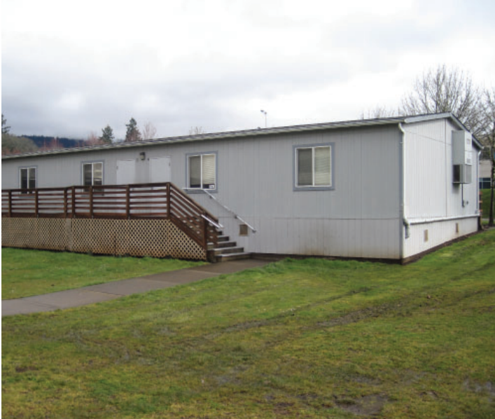
Chehalem Valley Middle School: Modular Classroom Facility
