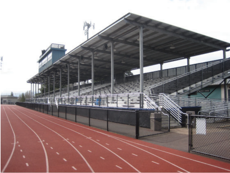
Newberg High School: Grandstand
