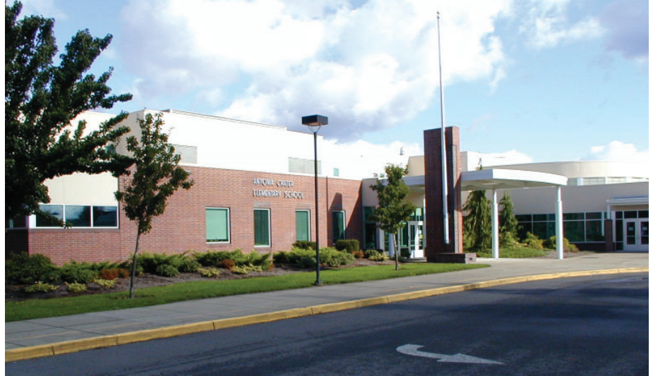
Antonia Crater Elementary School: Exterior View
