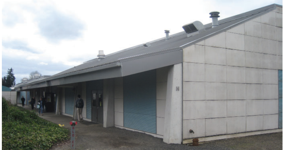
Newberg High School - Building H (CTE): Exterior View
