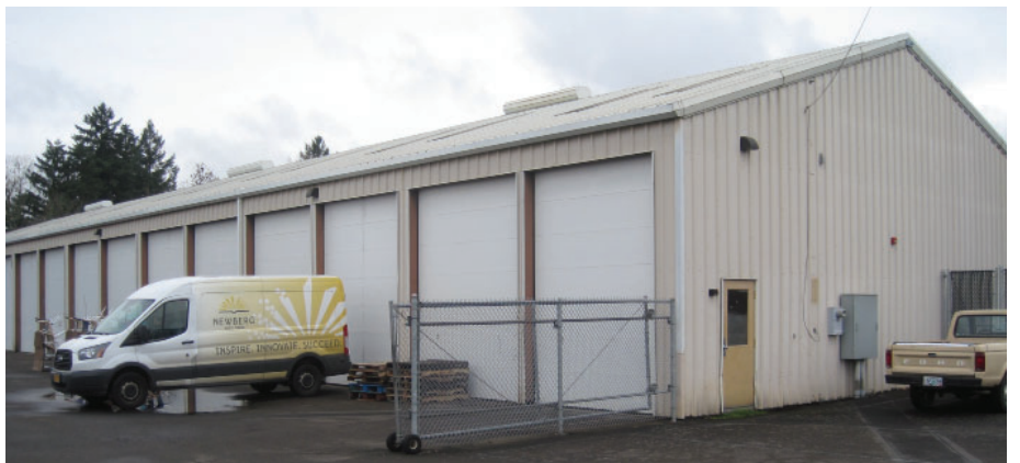
Physical Plant Building B: Exterior View
