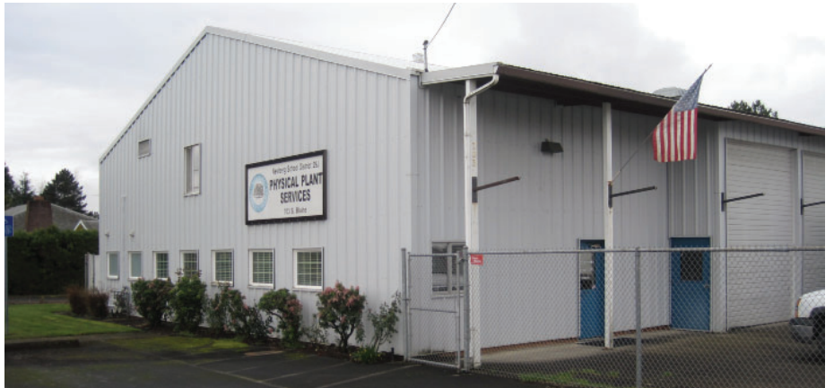
Physical Plant Building A: Exterior View
